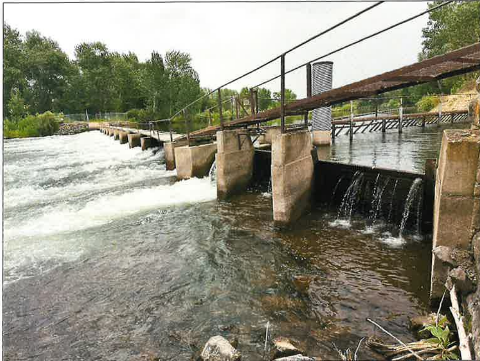
Photograph 5 (June 2024). Downstream of diversion structure with boards in place.
