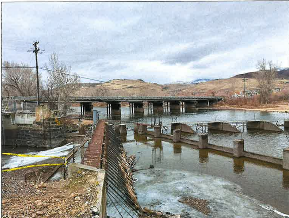
Photograph 6 (January 2025). Upstream of diversion structure looking at trashrack with no boards in place.
