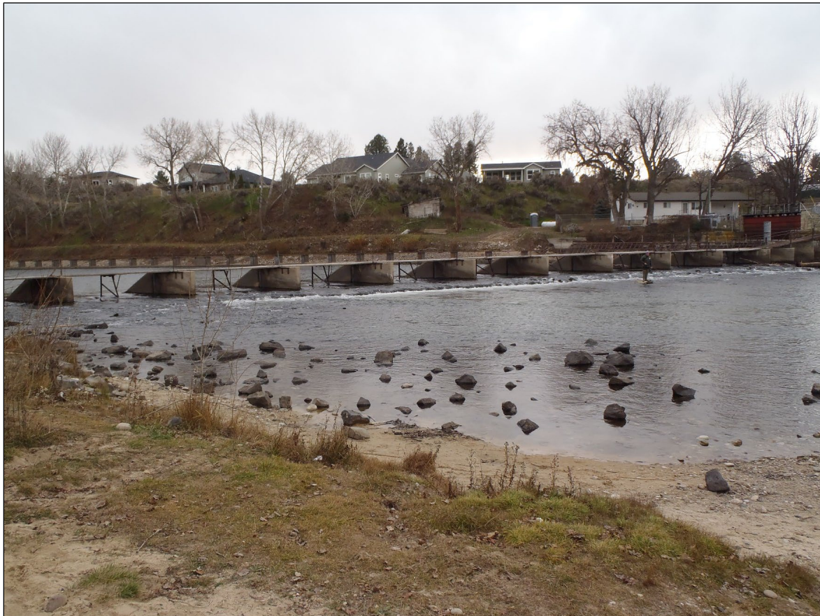
Figure 3.—Ridenbaugh Diversion without stop logs Installed (looking upstream).
