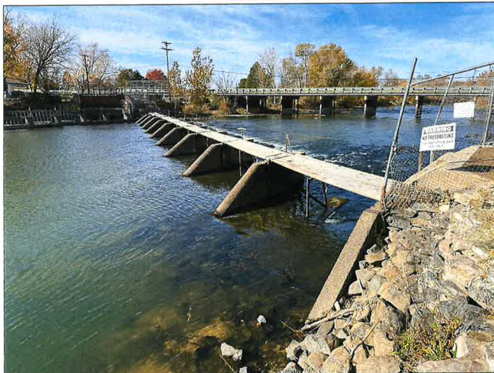
Photograph 4 (November 2023). Upstream of diversion structure with no boards in place.
