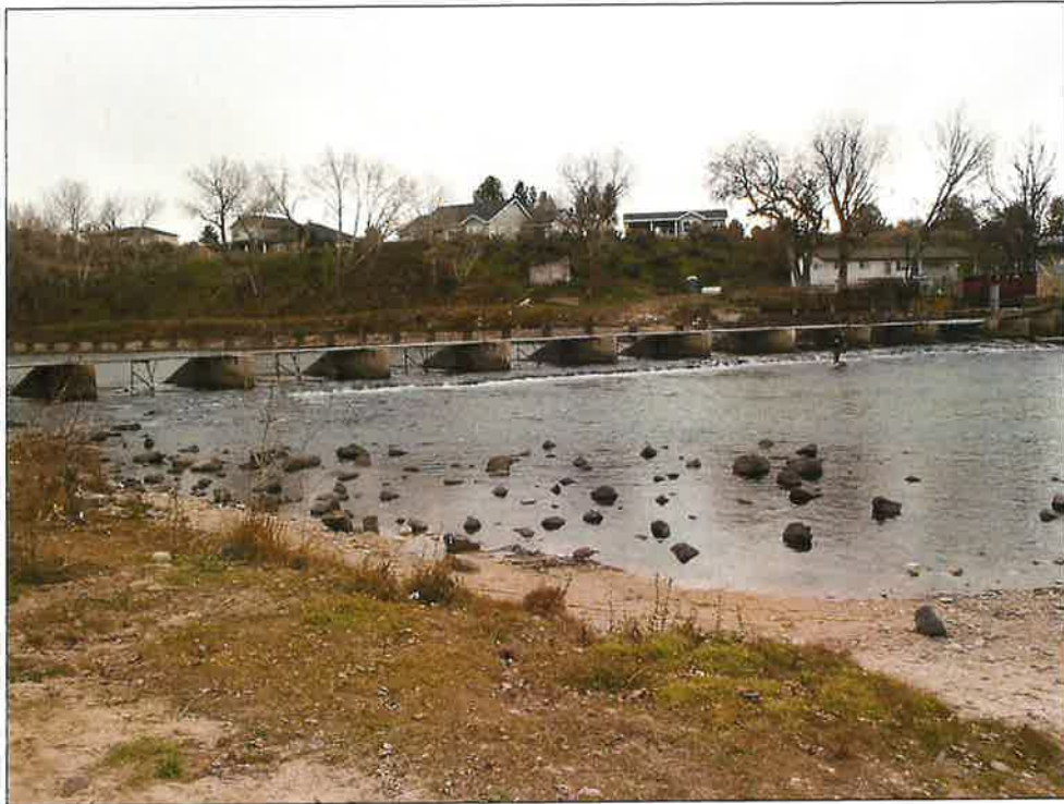
Photograph 1 (December 2023). Downstream of diversion structure with no boards in place.
