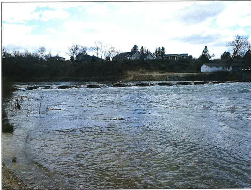
Photograph 3 (April 2025). Downstream of diversion structure with boards in place at 5,000 cfs.
