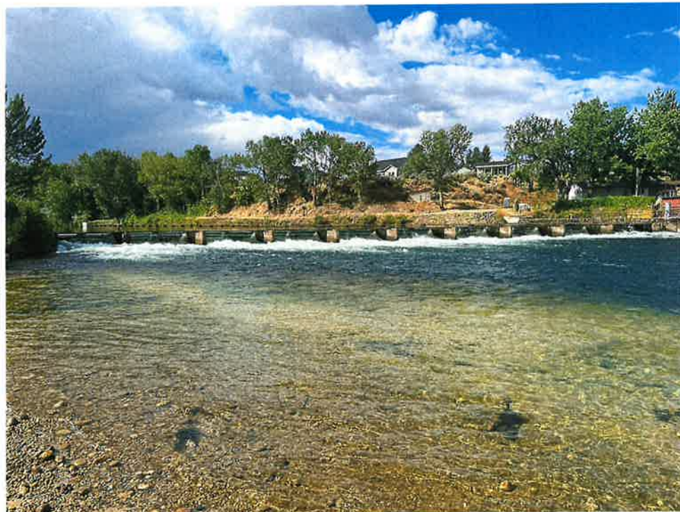
Photograph 2 (June 2024). Downstream of diversion structure with boards in place.
