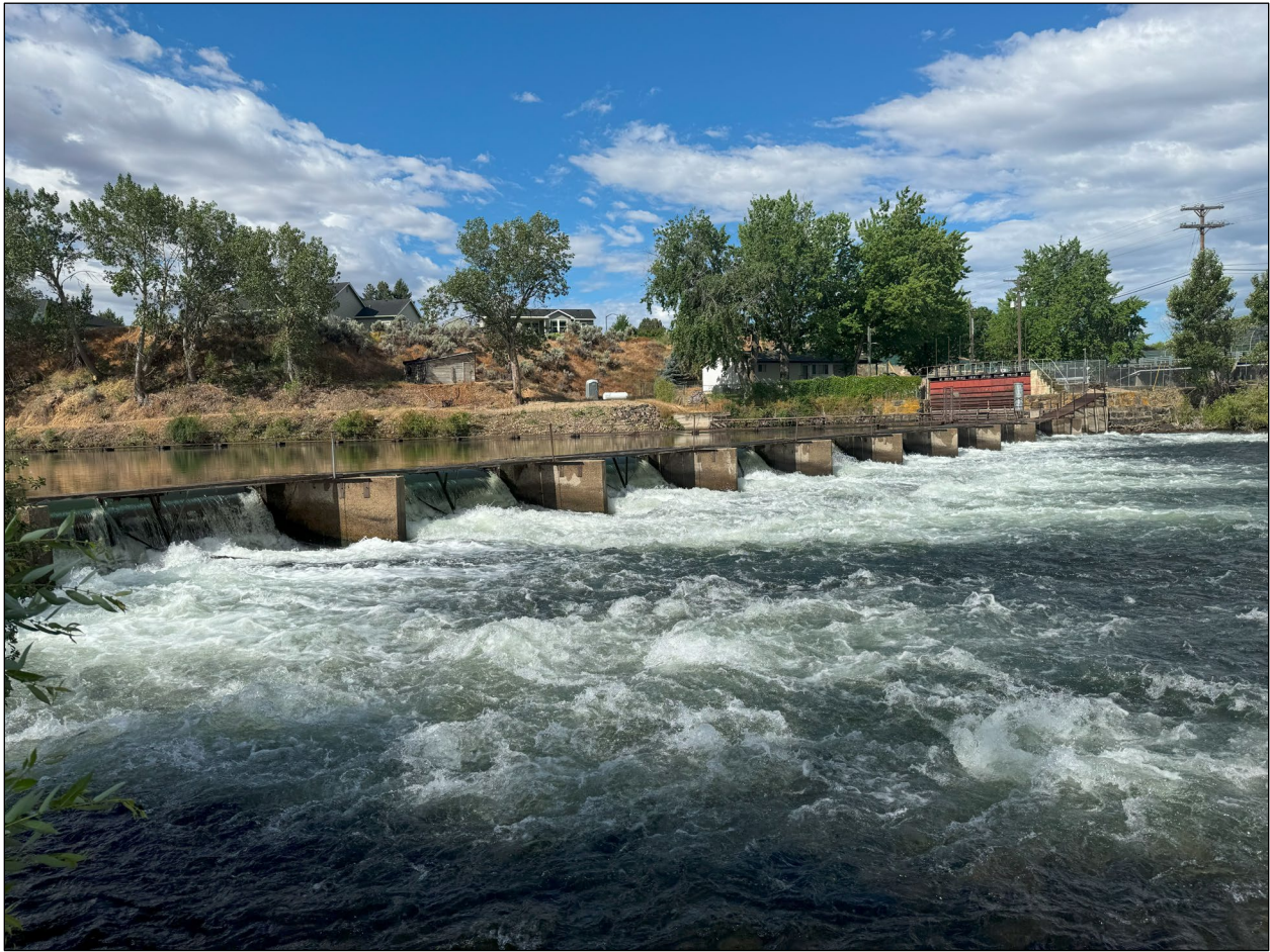
Figure 4.—Ridenbaugh Diversion with stop logs Installed (looking upstream).
