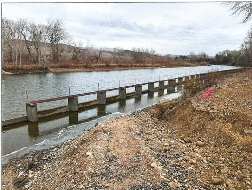
Photograph 8 (January 2025). Sediment wall with no boards in place at existing diversion structure.
